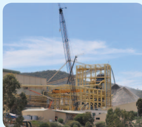
◀ The new ball mill at CVO will be one of the world’s most powerful, to grind Cadia East’s extra-hard ore.
